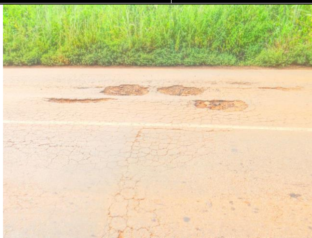
Figure 39 : Photo des fissurations transversales
